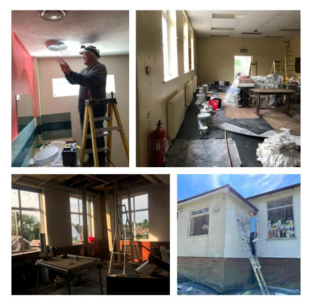
Our biggest challenge was electrical: how to make the Hall electrics safe, efficient and up to best in class modern standards. This involved systematically checking, replacing and repairing all of the electrical wiring in each of the Hall's rooms and open spaces, and all the outside electrical systems. We have ensured that the electrical works are safe, efficient and up to modern standards.
